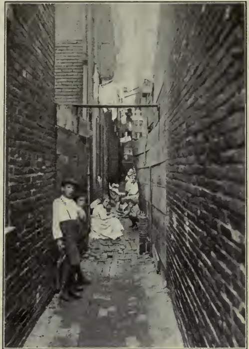
NARROW COURT BETWEEN DWELLING-HOUSES The court or alley is little more than 4 feet wide, and there were 7 houses (with 42 tenants) facing it when the photograph was taken.
